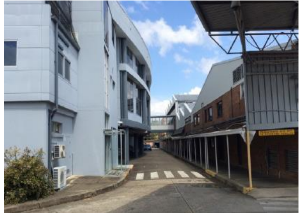
Figure 4. Existing industrial building
