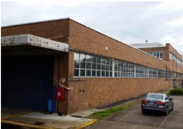
Figure 5. Existing industrial building
